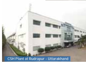
CSH Plant at Rudrapur - Uttarakhand
