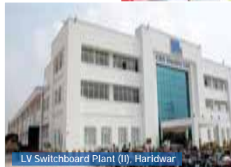
LV Switchboard Plant (II), Haridwar
