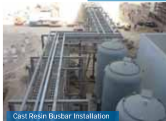
Cast Resin Busbar Installation
