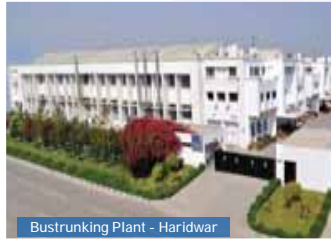
Bustrunking Plant - Haridwar
