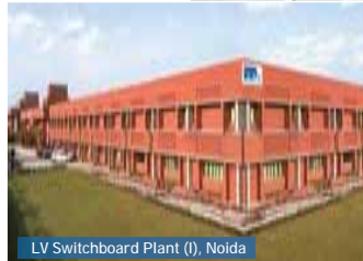
LV Switchboard Plant (I), Noida
