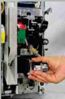
Mounting of Shunt trip
